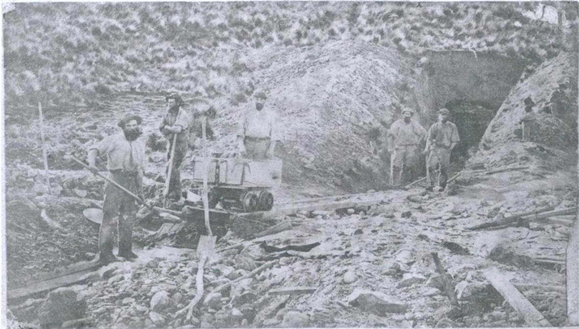
Gold mine sited near Waikaia / Switzers Museum
