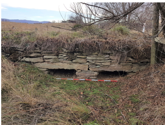
Plate 2. View north to stacked culvert (G41/595, GPS 376) beneath Ophir Bridge Road.
