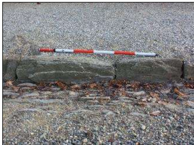
Plate 7. Example of schist slab kerbing and channelling, Rapid No 30 Swindon St, Ophir (Sarah Gallagher). View south.
