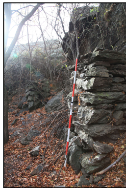
Plate ??. Stacked schist piers/plinths of water race pipeline/flume (G41/710, GPS 118). View north-west: M Sole).
