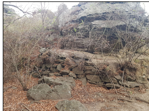
Plate ?. Stone stacking supporting the water race pipeline/flume around an outcrop (G41/710, GPS 118). View north-west: M Sole).
