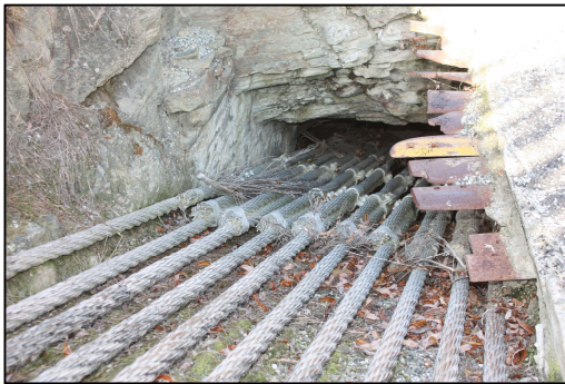
Plate 3. View to anchorings, Daniel O'Connell Bridge (G41/694, GPS 408). (Sarah Gallagher).
