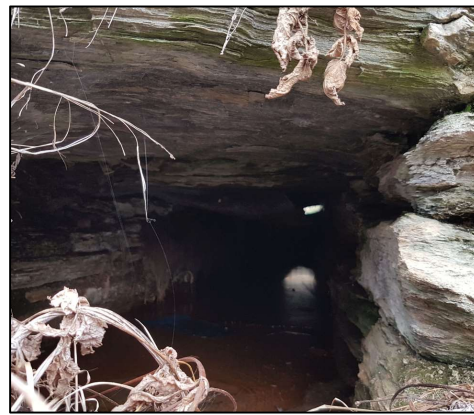
Plate 18. Stacked schist culvert (G41/575, GPS 375), Ophir Bridge Road. View south.
