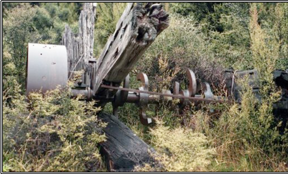
The collapsed stamp mill, showing one set of five cams.
