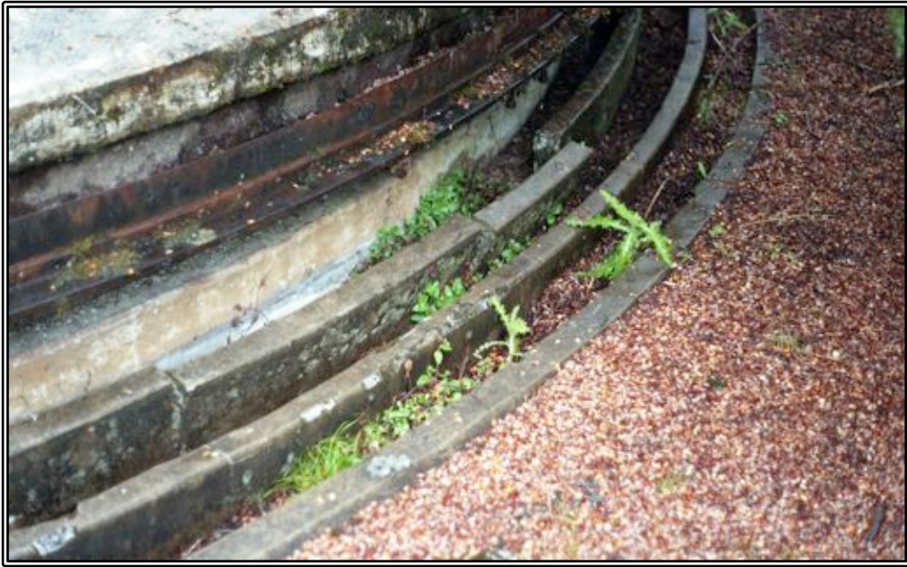
A detail of the peripheral drains of the buddle.
