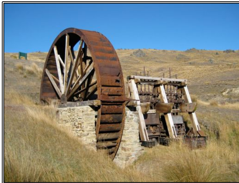
Figure 45 The Serpentine water wheel and battery (site H42/2). This wheel has been restored by the Department of Conservation.
