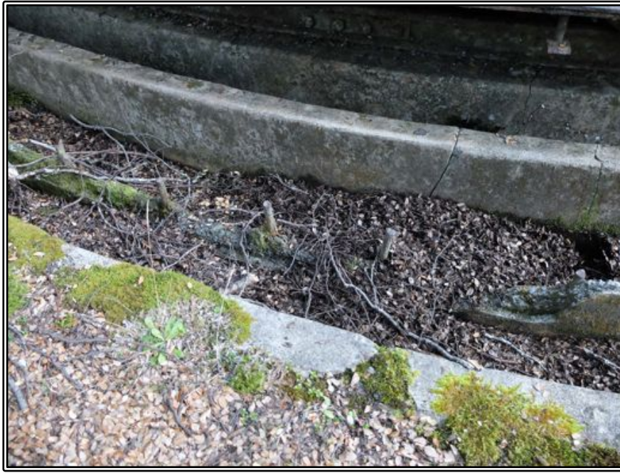
Figure 41 Deterioration of the cement channels in 2014, showing a section that has broken away exposing the reinforcing bars.
