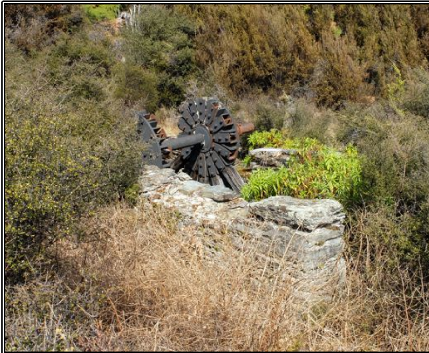
Figure 27 The Invincible water wheel in 2014. Note how all of the spokes at or above horizontal have now collapsed.
